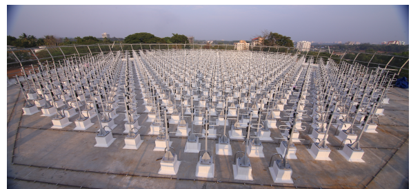
Figure 6. 619 element antenna array installed in the roof top
