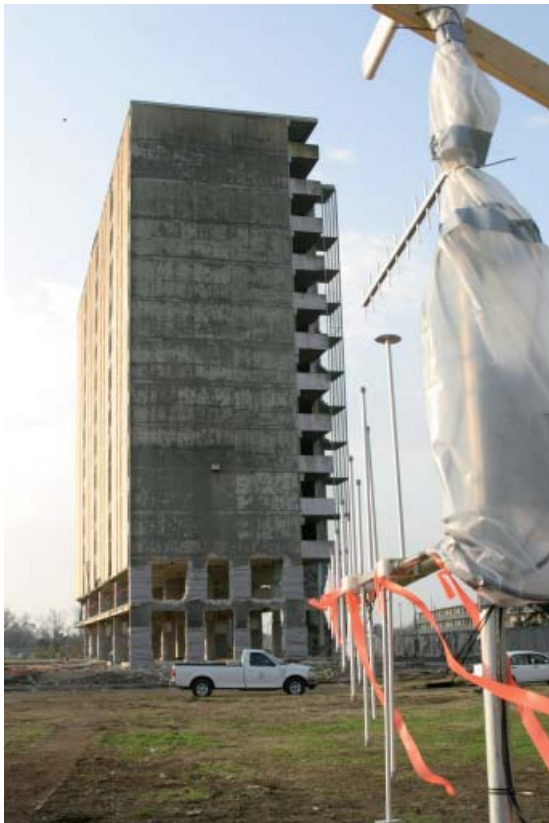
Figure 14a. A photo of the apartment building before the implosion.
