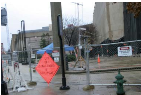
Figure 7a. The receiver site RX1 (northwest site) for the radio-mapping experiment for the convention center.
