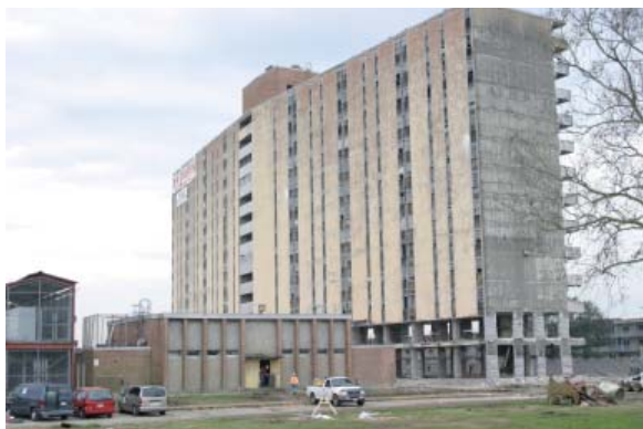
Figure 1a. A 13-story apartment building in New Orleans, Louisiana.
