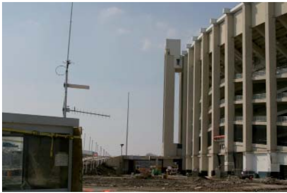
Figure 6a. The receiver site for the radio-mapping experiment for the sports stadium.
