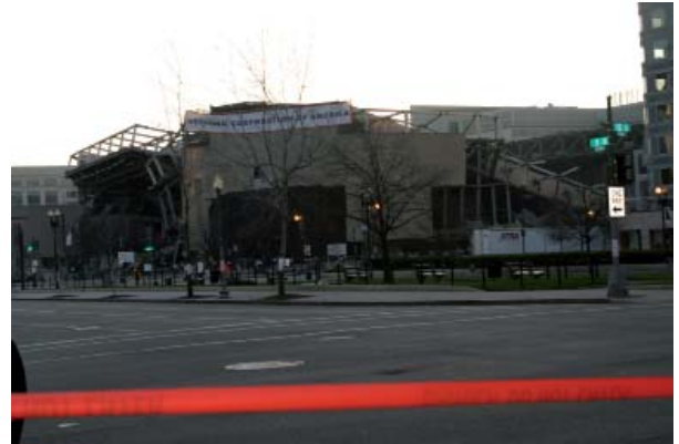
Figure 16b. A photo of the convention center after the implosion.
