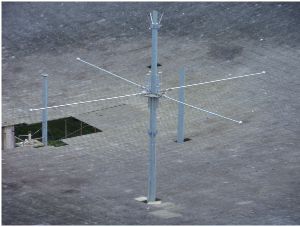
Figure 6. The first of six crossed-dipole HF feeds to be deployed on the Arecibo Observatory 305 m dish. These feeds will illuminate a wire subreflector, to be suspended from the towers that will in turn illuminate the dish. Three feeds are sized for 5.1 MHz ( \lambda = 58.8 m) and three feeds are for 8.175 MHz ( \lambda = 36.7 m). Modeling of the configuration suggested a 22.2 dBi one-way gain at 5.1 MHz ( \sim 12^\circ FWHM beamwidth), and a 25.5 dBi gain at 8.175 MHz ( \sim 8^\circ FWHM beamwidth). As six 100 kW CW transmitters are available, each polarization of each of the three feeds at a single frequency will be separately driven, permitting full polarization flexibility. The transmitters are class-A. However, pseudo-pulsed operation will be possible. Later operations at 3.175 MHz may become possible ( photo July 21, 2013, JDM).
