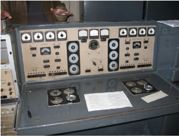
Figure 4. The 32-m antenna drives are still partially controlled with the old (vacuum-tube-based) steering system (photo: Gudmund Wannberg).
