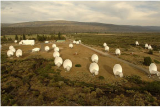
Figure 11. Part of the ATA-42 array that is now operational at Hat Creek Radio Observatory in Northern California. The hydro-formed 6.1 m diameter dishes use a Gregorian-optics configuration (with ground shield), incorporating the wideband pyramidal feed shown in Figure 8.
