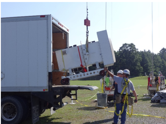
Receiver on Crane Hoist
