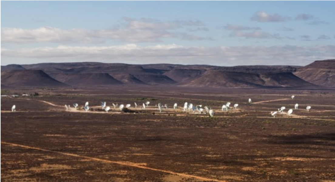
An aerial view of the inner core of the MeerKAT telescope. About 54 of the 13.5-meter antennas lie within the 1 km diameter core.
