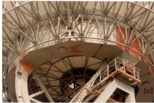
Figure 8. The 32-m Merlin telescope of the Jodrell Bank Observatory in Cambridge, UK. The reflector backup structure is connected to the ring girder at four positions 45° from the elevation bearings by flexures, visible in the middle of the detail picture (two nodes to the left of the red painted area) (H. Kärcher).
