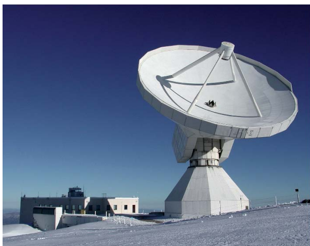
Figure 12. The 30-m millimeter radio telescope (MRT) of IRAM at 2850 m altitude in the Sierra Nevada of southern Spain. Completely wrapped in thermal insulation and with active control of the temperature of the structure, it operates down to a wavelength of 0.8 mm (J. Baars, IRAM).
