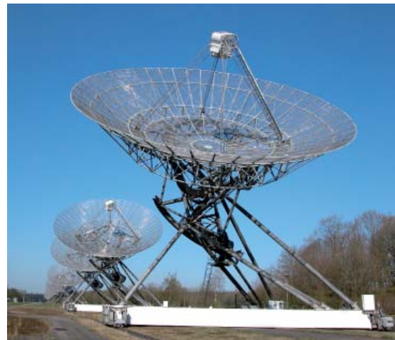
Figure 7. The Westerbork Synthesis Radio Telescope, with 14 polar-mounted 25-m antennas. Through the mesh surface, the declination cradle can be seen providing the four-point support for the reflector's structure and the quadripod. The circular gear-racks provide the movement in hour angle and declination. The two antennas in front can take any position on a 300 m-long rail track. The other fixed antennas are 144 m apart (ASTRON).
