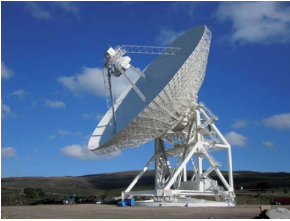
Figure 30. The 64-m diameter Sardinia Radio Telescope (SRT) (INAF).
