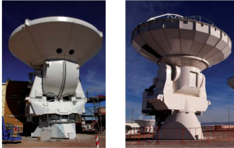
Figure 25. (a) The European ALMA antenna, delivered by consortium AEM. (b) The US antenna, produced by Vertex. In both, the carbon-fiber-reinforced plastic reflector backup structure is shielded against solar radiation by outside cladding. Steel parts of the yoke and base are covered with thermal insulation. The reflector diameter is 12 m and the surface precision is about 20 \mu\text{m} rms (ALMA-ESO/NOAJ/NRAO).
