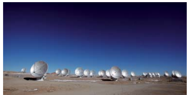
Figure 29. About one-third of the ALMA array at 5000 m altitude on the Llano de Chajnantor in the Atacama Desert of northern Chile. The main instrument consists of 50 antennas of 12 m diameter and is supplemented by the Atacama Compact Array (ACA) of 12 antennas of 7 m diameter (in the right background of the picture), plus four more 12 m antennas (ALMA-ESO/NAOJ/NRAO, C. Padilla).
