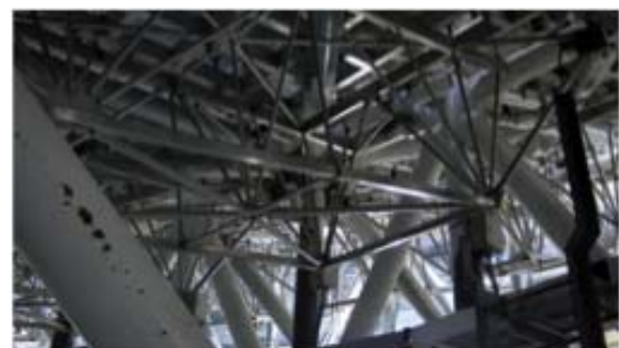
Figure 22b. A rear view of a panel unit installed in the backup structure of the LMT. The segments of about 5 m size are supported at their corners on the backup structure by motorized adjusters.
