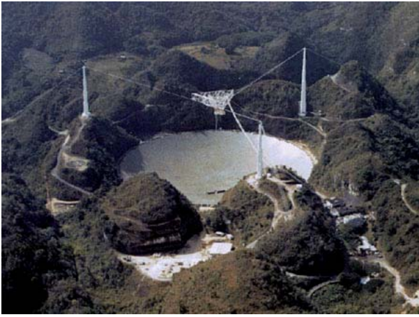
Figure 1. The Arecibo radio/radar telescope. It was constructed in the early 1960s, dedicated in late 1963, and commissioned in 1964. The reflector surface diameter is 1000 feet (305 m). Note that the antenna beamwidth at 70 cm wavelength (430 MHz) is 10 arc-minutes, and 1.8 arc-minutes at 13 cm wavelength. The moon’s angular width is 30 arc-minutes to 33 arc-minutes.
