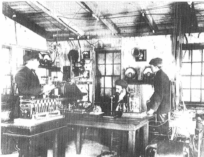
Inside the Brant Rock Radio Shack: Operators in transmitting position.
