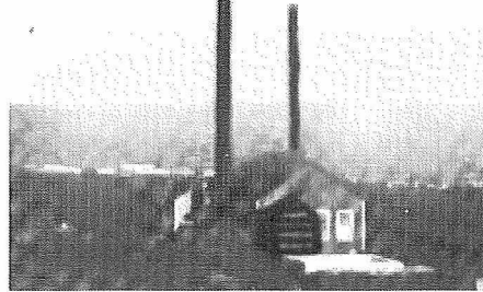
Photo 5. The Brant Rock, Massachusetts, tower, with the radio shack at the bottom. The tall pipe extending above the transmitter building is the smoke-stack for the steam engine, which was used (belt drive) to drive the AC generator for Fessenden's synchronous, rotary spark gap telegraphy transmitter and, later, his HF alternator for telegraphy and telephony.
